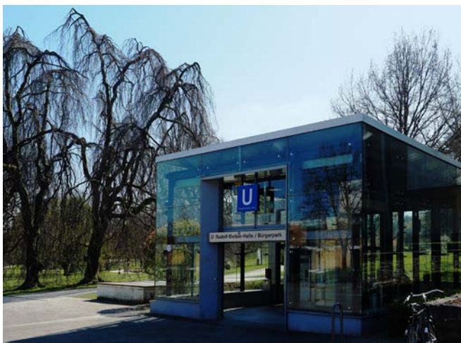
Eingang U-Bahn Station Oetkerhalle (Foto: Peter Wolf)
